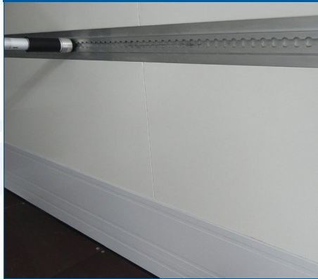
recessed in the walls
